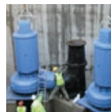
IRELAND Maintaining pressure at pumping stations
